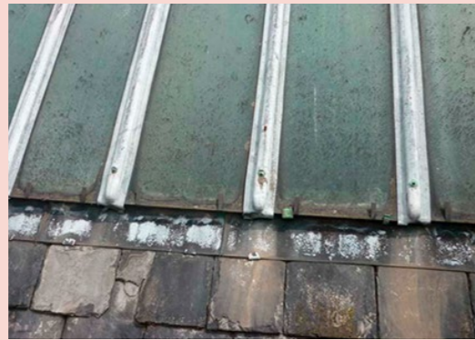
Fig. 53 / Welsh slates and roof lights in poor condition [Source: Hereford Library Condition Survey 2010, p.42 CMP]
